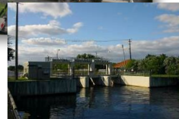
G-54 Structure (Sewell Lock) and flooding in Ft. Lauderdale 2020.
